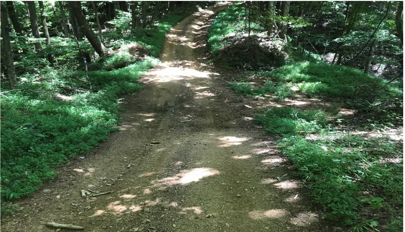
Figure 08 (Low spot in trail. Sediment flows down slope; 37^{\circ}15'49''\text{N} , 82^{\circ}07'43''\text{W} )
