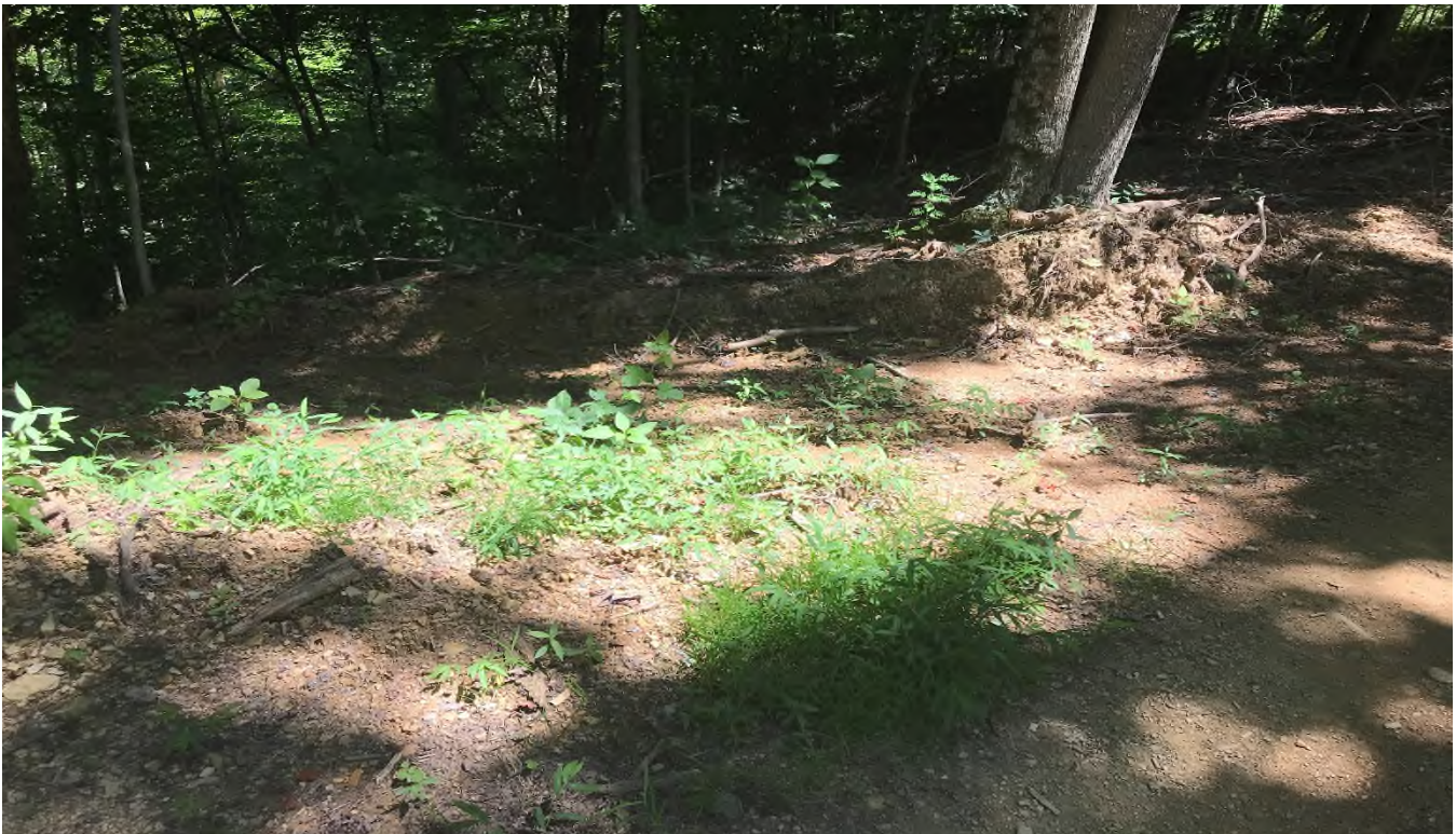
Figure 06 (Window cut on section of trail construction shown in Figures 4 and 5 sending concentrated flows over the slope; 37°16'05"N, 82°08'11"W)
