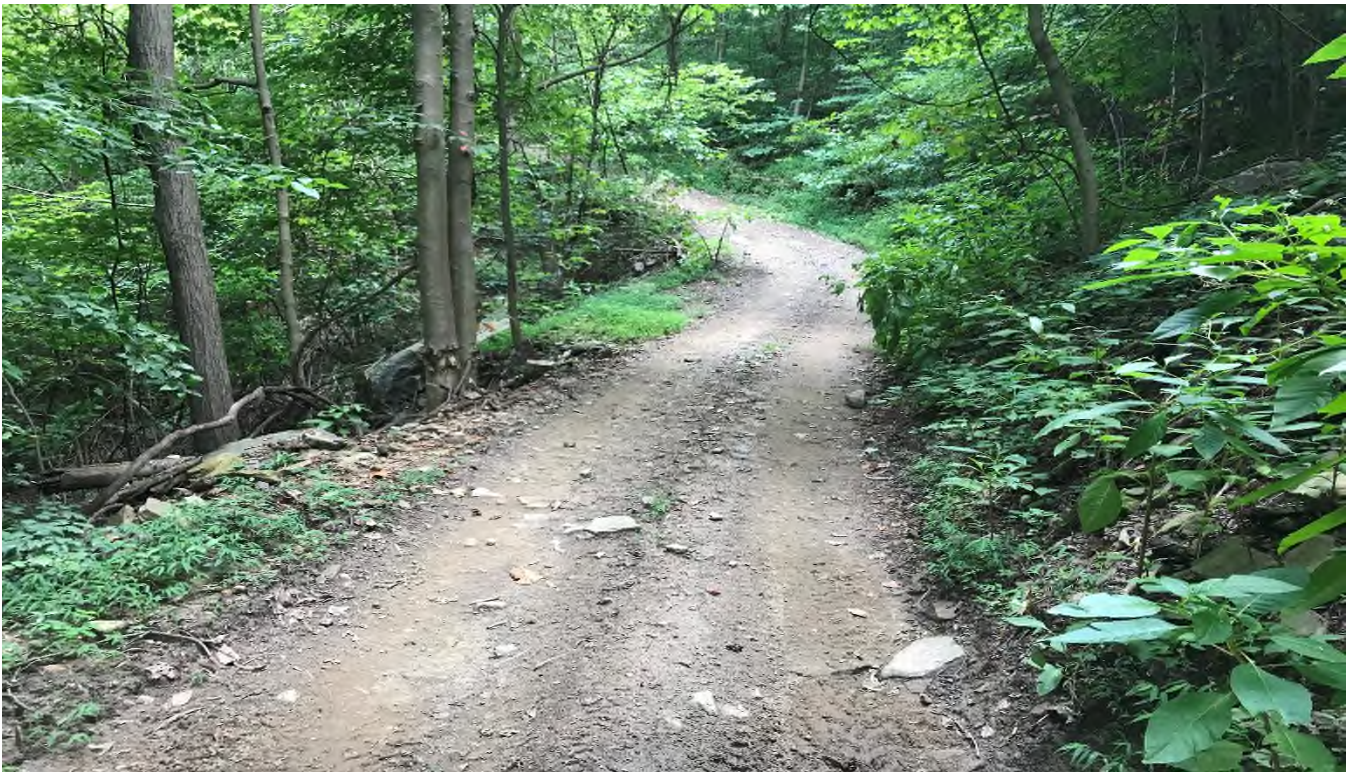
Figure 21 (Concentration of flows from the trail. Flows discharging over the slope resulting in sediment loss shown in Figure 22; 37°16'50"N, 82°06'53"W)
