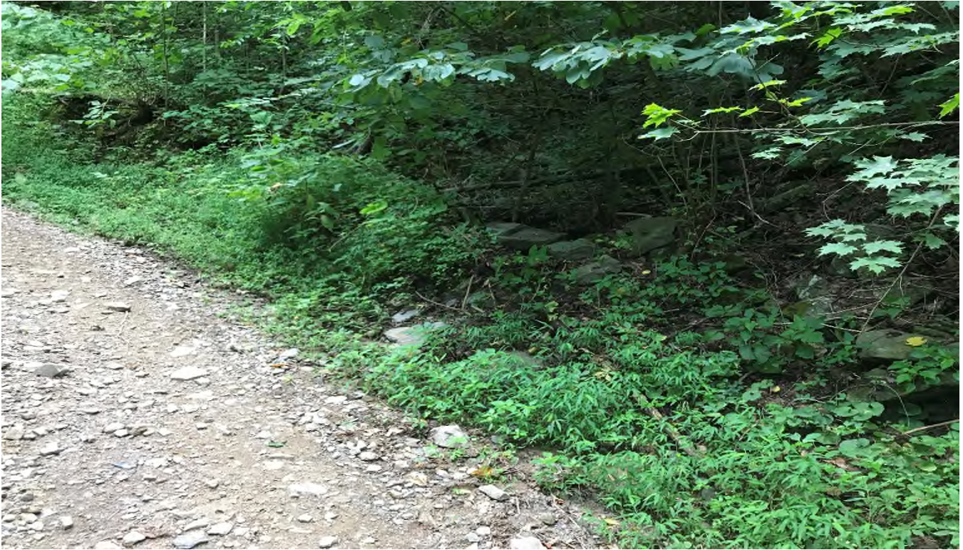
Figure 23 (Natural hollow crossed by trail with no visible cross pipe. Natural drainage intercepted by trail and conveyed down gradient away from hollow; 37°16'50"N, 82°06'53"W)
