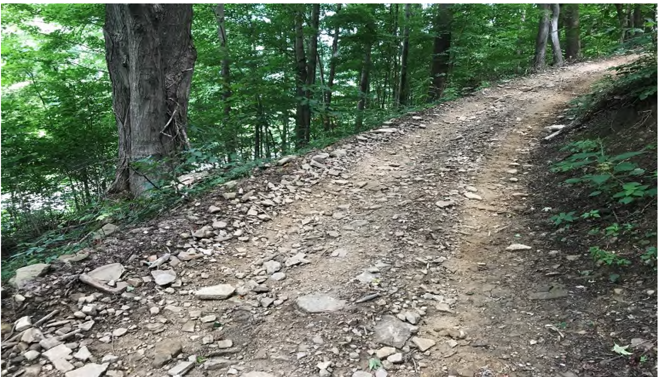
Figure 20 (Trail concentrating flows down the slope leading to the area shown in Figure 19 above; 37°16'52"N, 82°06'55"W)
