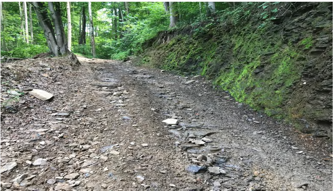
Figure 16 (New land disturbance associated with either new trail construction or widening of an existing trail. Photo taken facing uphill away from the entrance shown in Figure 11 above; 37°16'52"N, 82°06'57"W)
