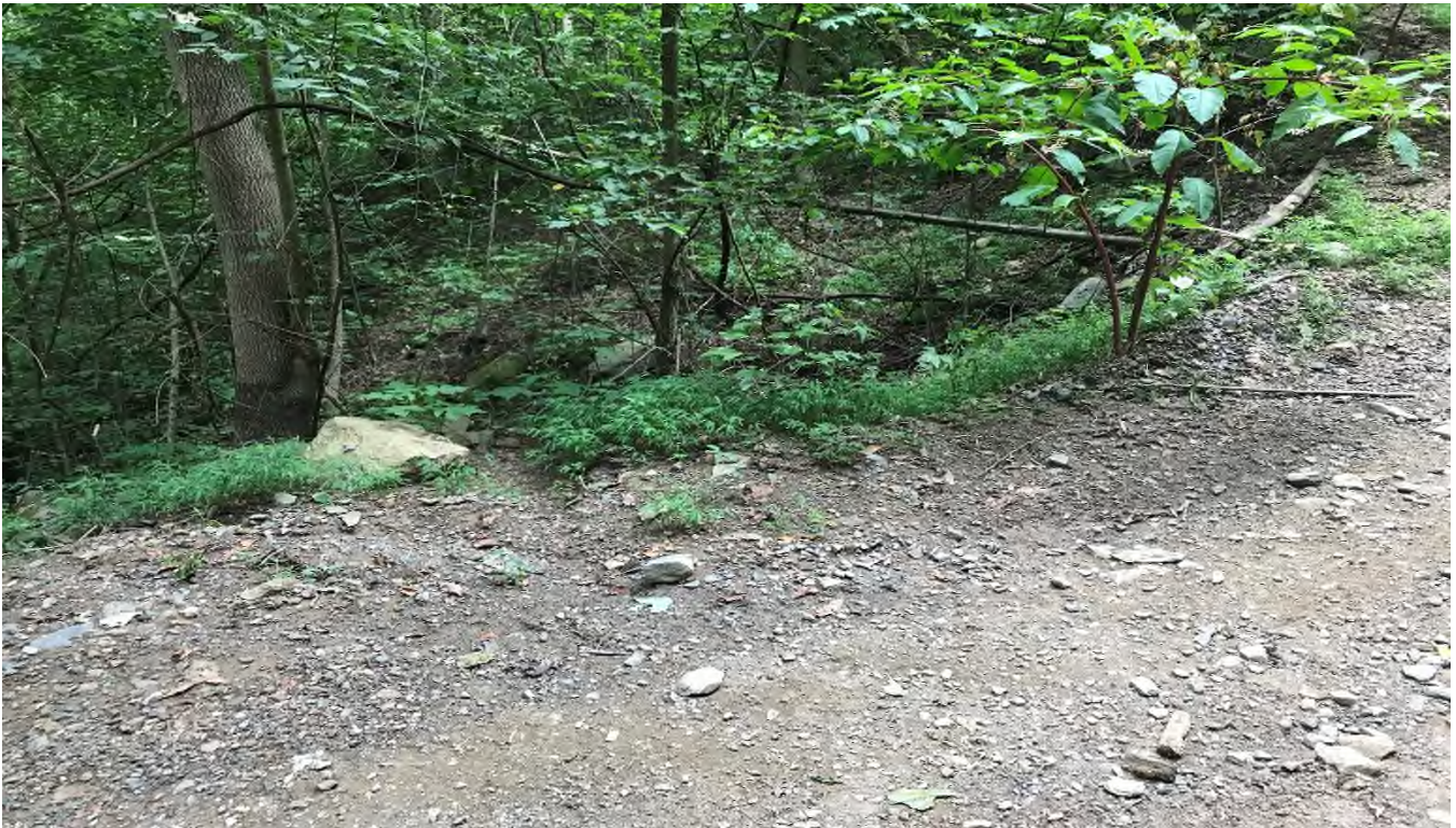
Figure 24 (Out slope of trail down gradient of natural drainage shown in Figure 23; 37°16'50"N, 82°06'53"W)
