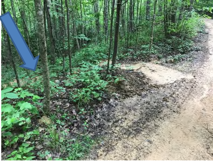
Fig. 27 Description: Off-site Sediment Loss onto down gradient properties from trail erosion due to the lack of sediment trapping controls
