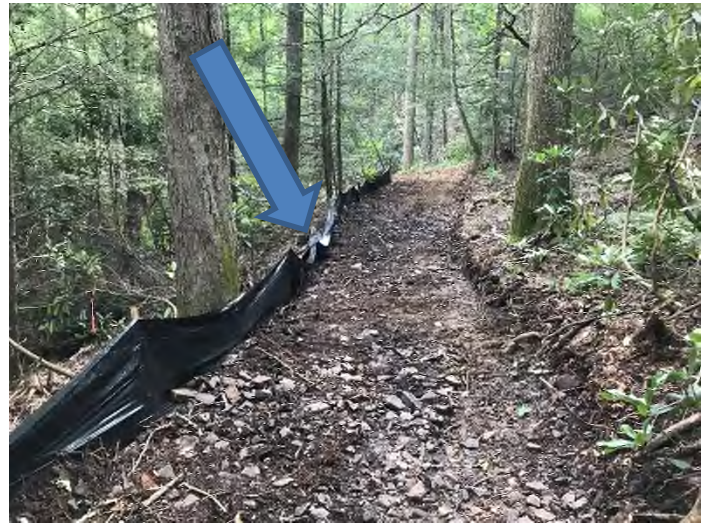
Fig. 4 Description: Silt fence not maintained
