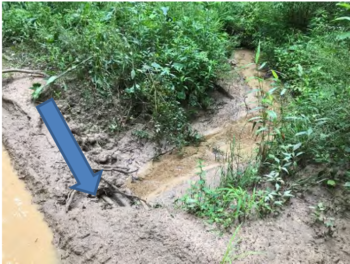
Fig. 23 Description: Culvert installation without appropriate permits, culvert not countersunk, and no outlet protection
