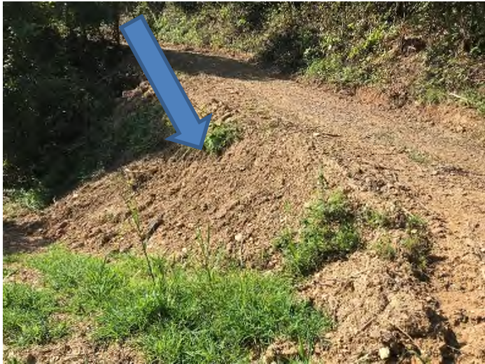
Fig. 5 Description: Stabilization timeframes exceeded
