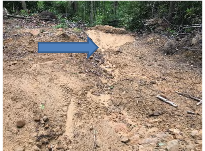
Fig. 14 Description: Concentrated stormwater runoff not directed to an adequate receiving channel or converted to sheet flow
