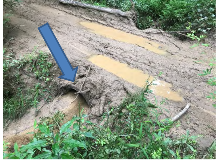
Fig. 24 Description: Culvert installation without appropriate permits, culvert not countersunk, and no outlet protection
