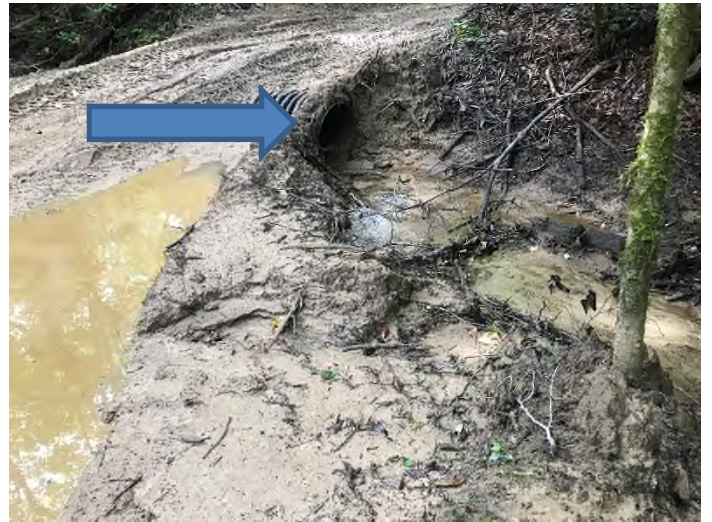
Fig. 24 Description: Culvert installation without appropriate permits, culvert not countersunk, and no outlet protection
