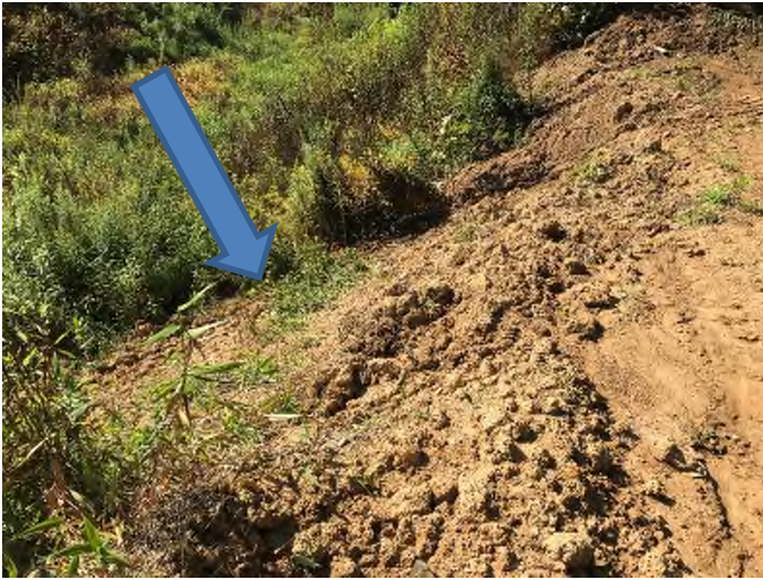
Fig. 3 Description: Silt fence not maintained
