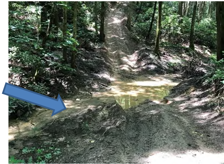
Fig. 31 Description: Sediment impacts to potential jurisdictional stream due to trail erosion from perpetual riding, lack of sediment trapping controls, and lack of stabilization
