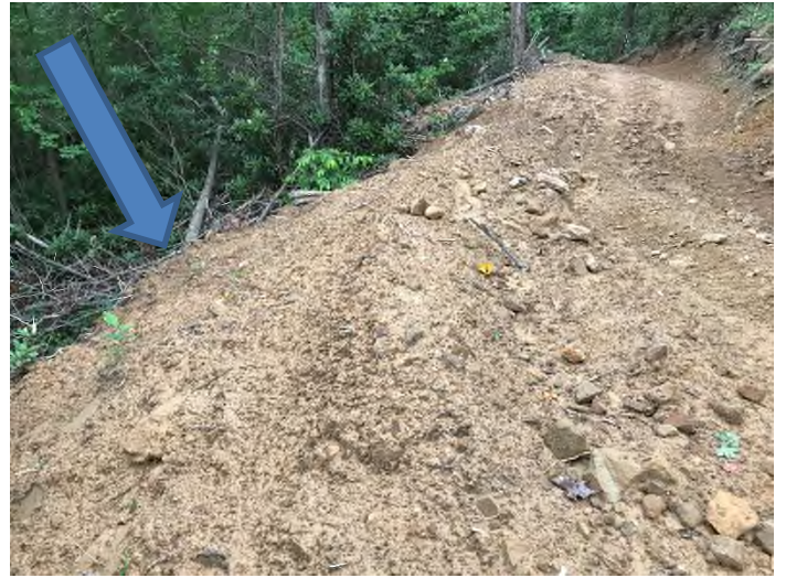
Fig. 4 Description: Silt fence not maintained
