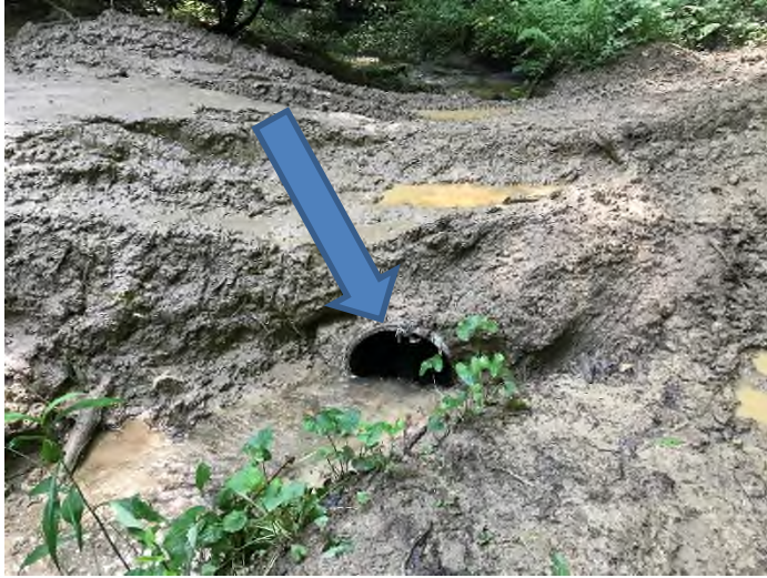
Fig. 23 Description: Culvert installation without appropriate permits, culvert not countersunk, and no outlet protection
