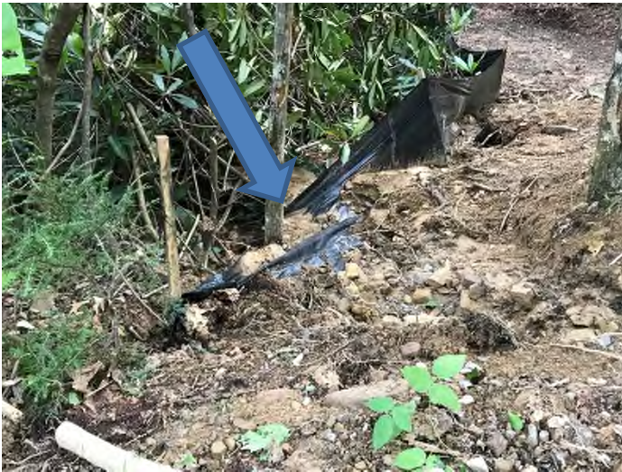
Fig. 3 Description: Silt fence not maintained
