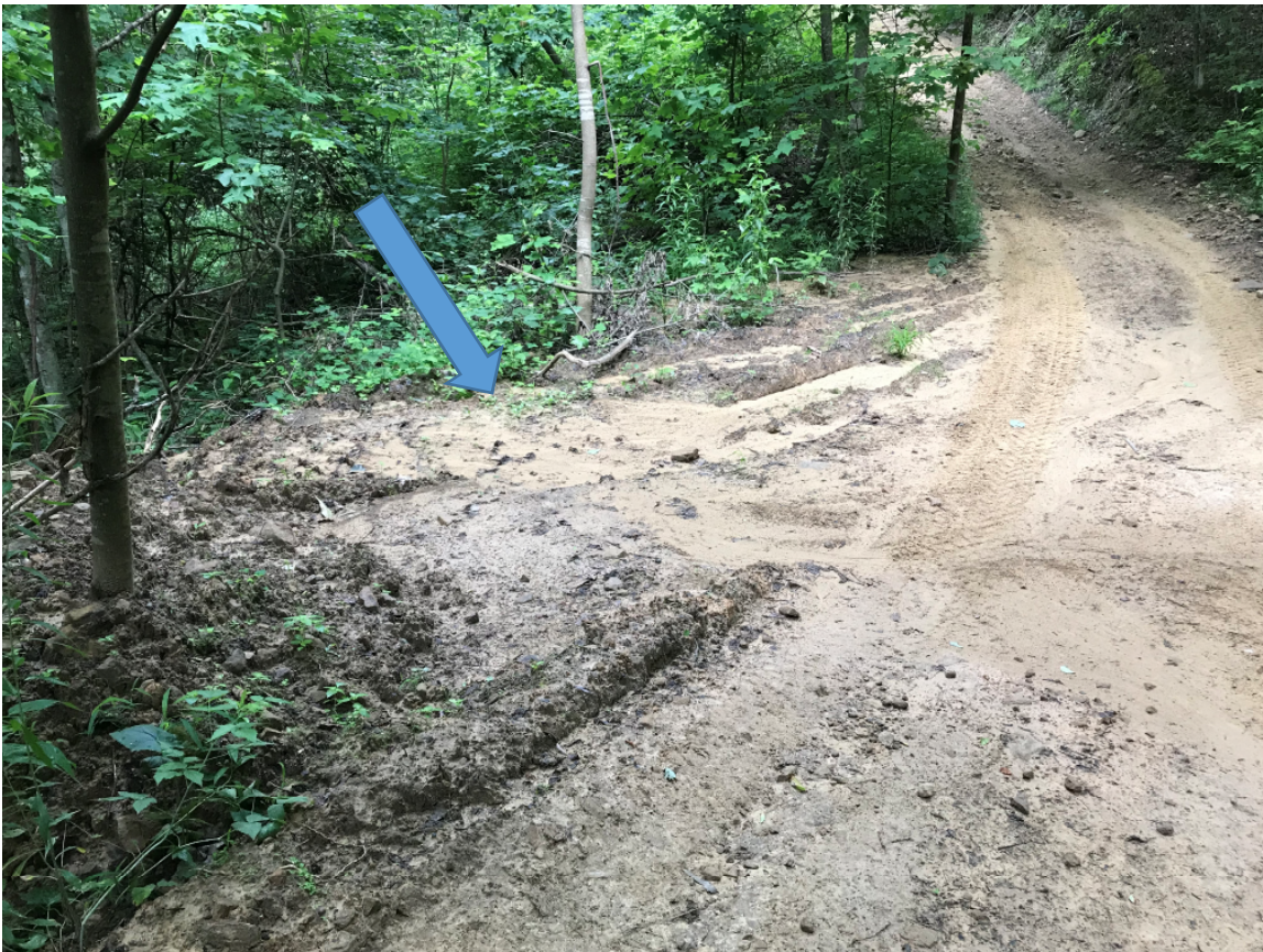
Figure 46 (Section of Trail 16 with a cut allowing unfiltered runoff from the trail to discharge over the slope into a drainage swale leading to Curran Branch; 37.29801° , -81.39059° )
