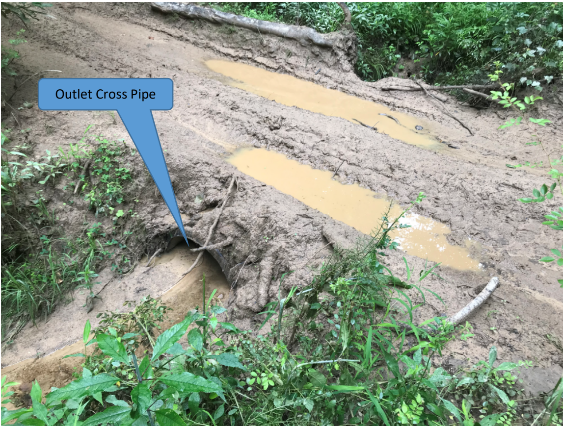
Figure 50 (Cross pipe in Curran Branch on a Section of Trail 67 and sediment deposition observed in Curran Branch from unfiltered runoff from the trail; 37.29746°, -81.39559° )
