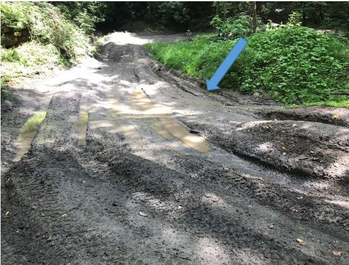
Figure 22 (Trail 14 crossing wet hollow which discharges to Haynes Branch with sediment deposition observed down gradient; 37.29584° , -81.37292° )
