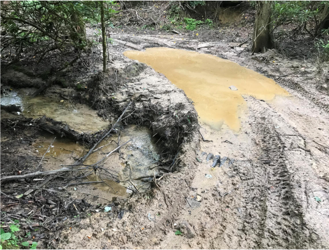
Figure 56 (Section of Trail 67 with a cut allowing unfiltered runoff from the trail to discharge over the slope into a drainage swale leading to Curran Branch; 37.29464°, -81.39353° )
