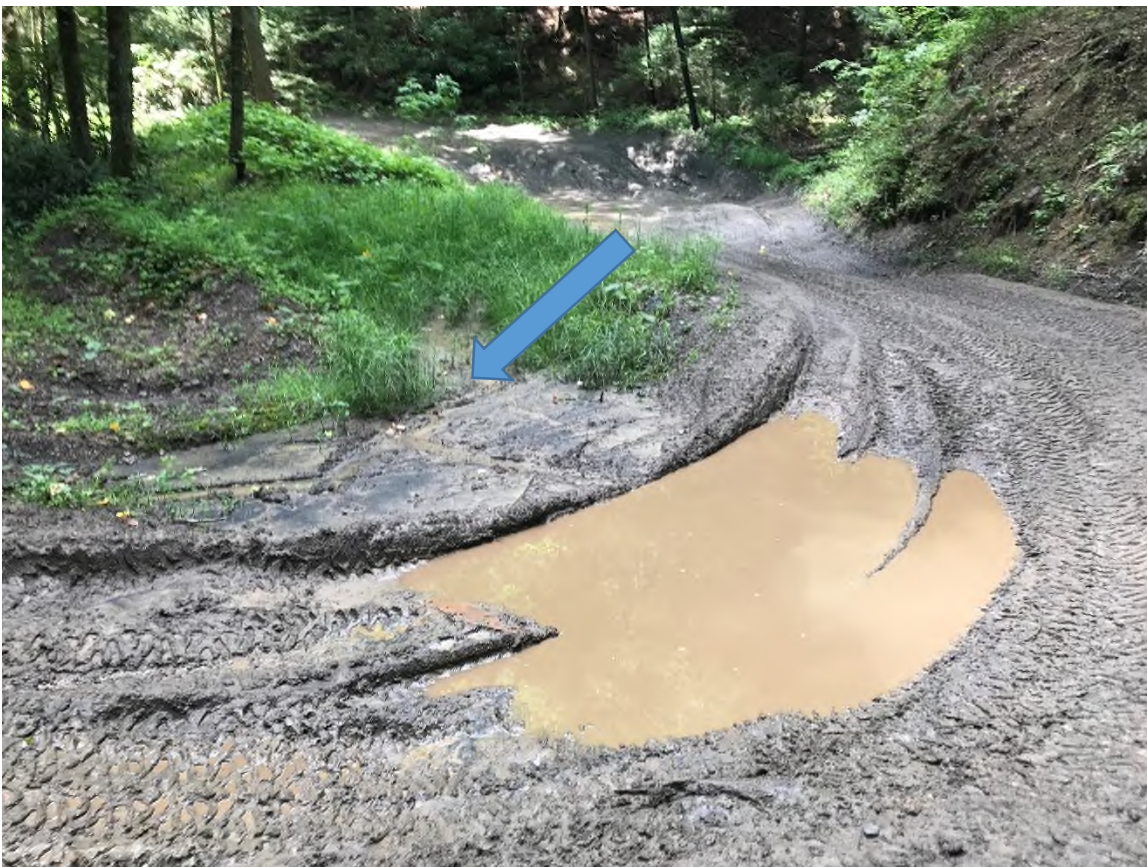
Figure 22 (Trail 14 crossing wet hollow which discharges to Haynes Branch with sediment deposition observed down gradient; 37.29584° , -81.37292° )
