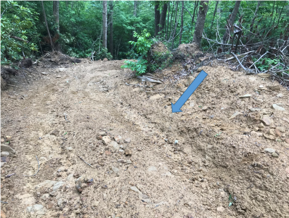
Figure 60 (Section of Trail 67 with a cut allowing unfiltered runoff from the trail to discharge over the slope into a drainage swale leading to Curran Branch; 37.29477° , - 81.39217° )
