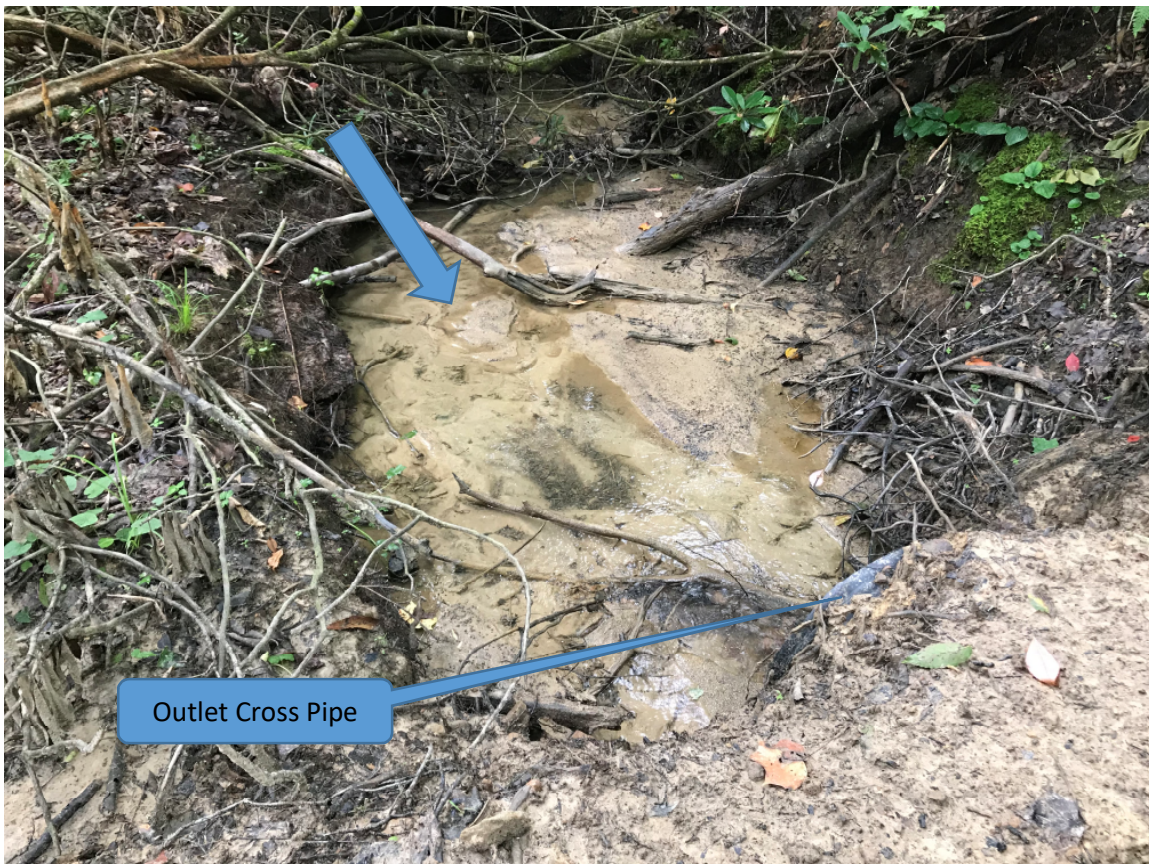
Figure 54 (Cross pipe in Curran Branch on a Section of Trail 16 and sediment deposition observed in Curran Branch from unfiltered runoff from the trail; 37.29664° , -81.39494° )
