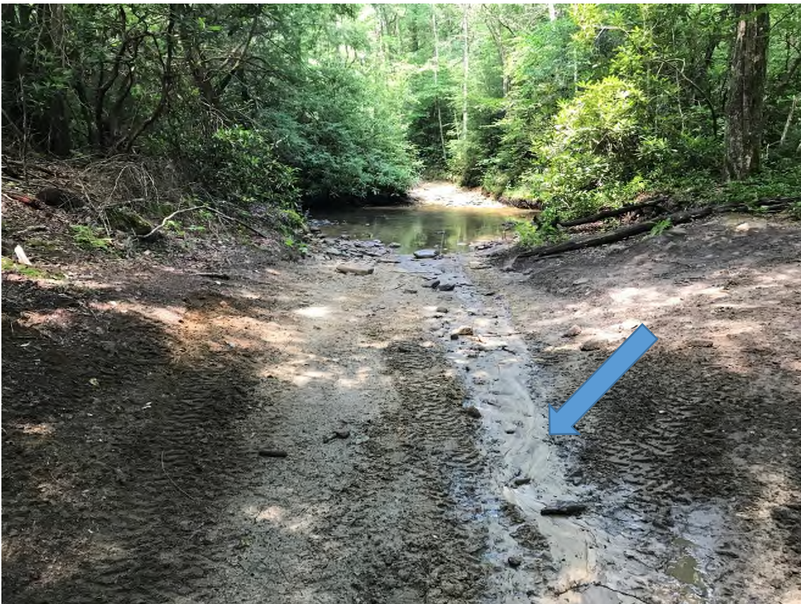
Figure 18 (Trail 14 crossing Laurel Fork with a trail of sediment observed leading to Laurel Fork; 37.29433° , -81.37004° )
