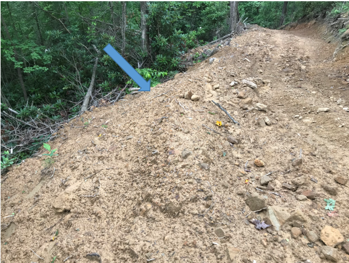
Figure 58 (Un-stabilized land disturbance from what appeared to be a newly constructed section of Trail 67 with trail erosion and sediment deposition observed down gradient; 37.29461°, -81.39249° )
