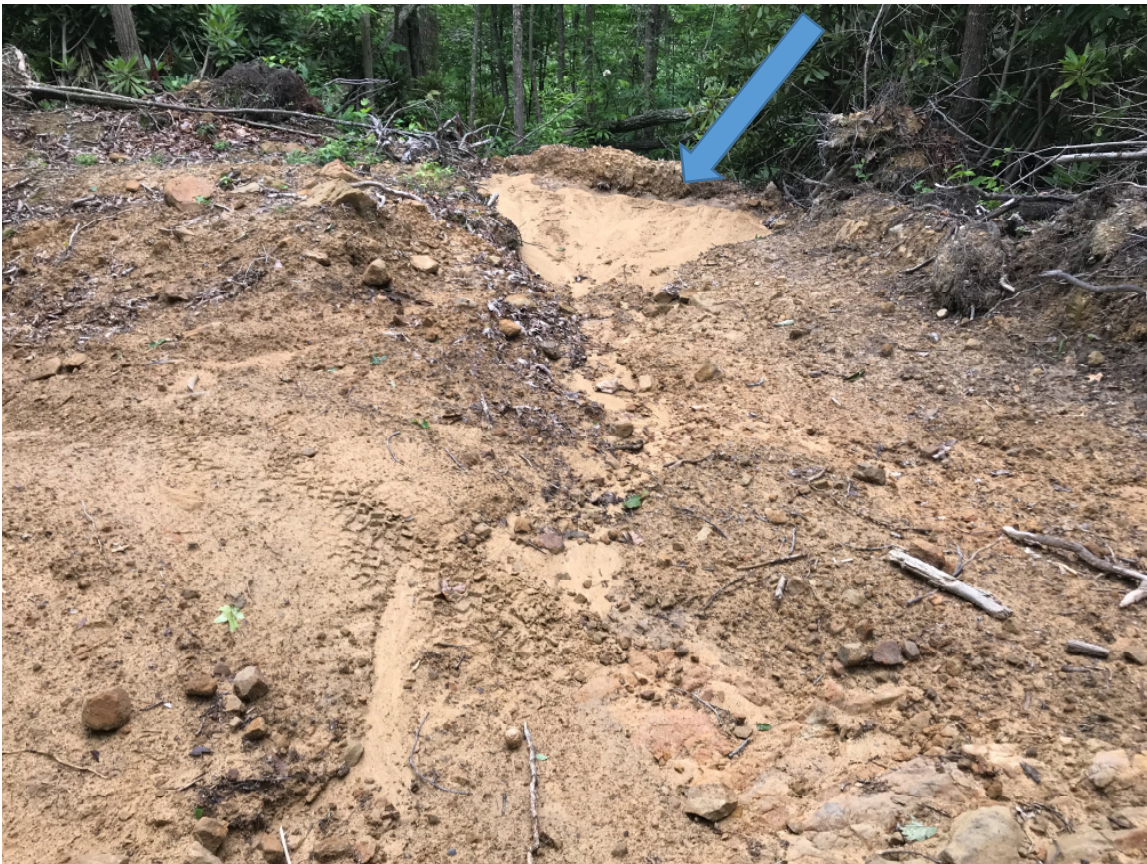
Figure 60 (Section of Trail 67 with a cut allowing unfiltered runoff from the trail to discharge over the slope into a drainage swale leading to Curran Branch; 37.29477° , - 81.39217° )
