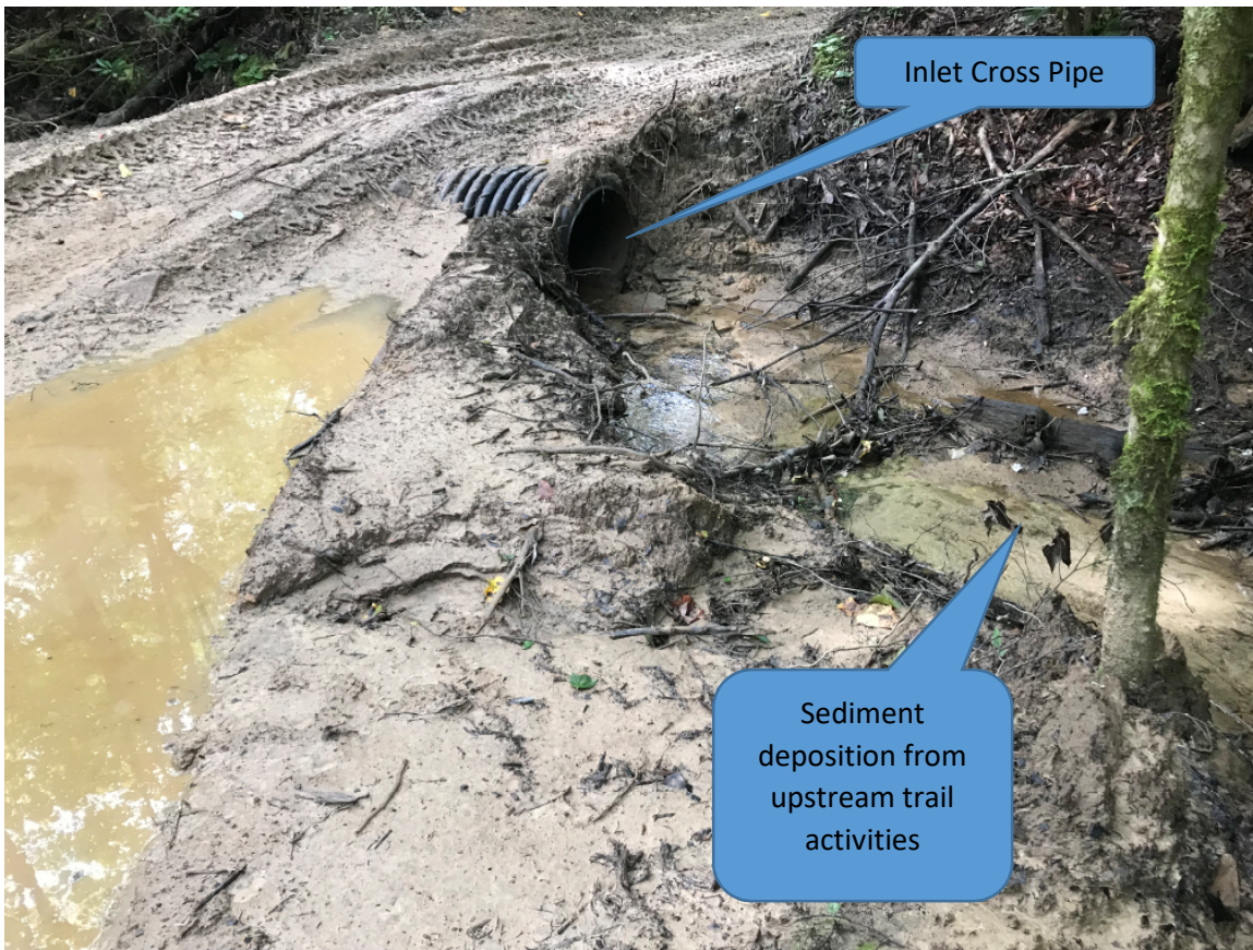
Figure 54 (Cross pipe in Curran Branch on a Section of Trail 16 and sediment deposition observed in Curran Branch from unfiltered runoff from the trail; 37.29664° , -81.39494° )
