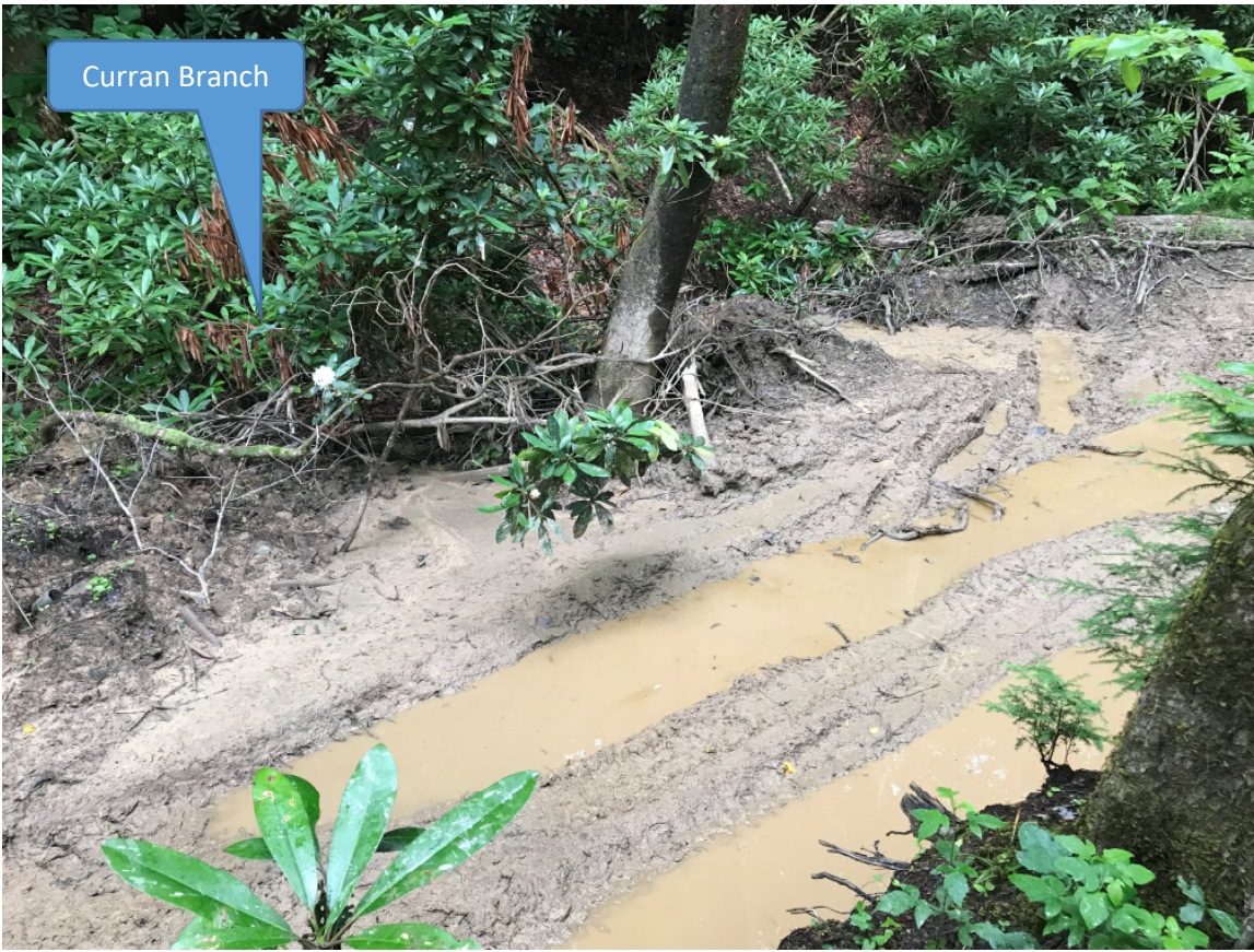
Figure 48 (Cross pipe in Curran Branch on a Section of Trail 67 and sediment deposition observed in Curran Branch from unfiltered runoff from the trail; 37.29746° , - 81.39559° )
