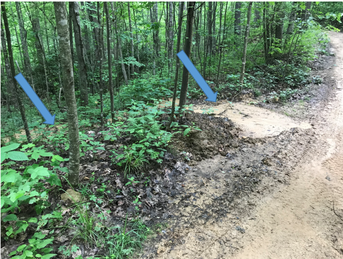
Figure 44 (Section of Trail 16 with a cut allowing unfiltered runoff from the trail to discharge over the slope into a drainage swale leading to Curran Branch; 37.29713° , -81.39059° )
