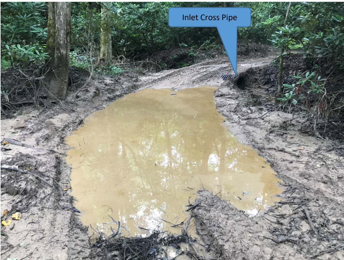
Figure 52 (Cross pipe in Curran Branch on a Section of Trail 16 and sediment deposition observed in Curran Branch from unfiltered runoff from the trail; 37.29664°, -81.39494° )
