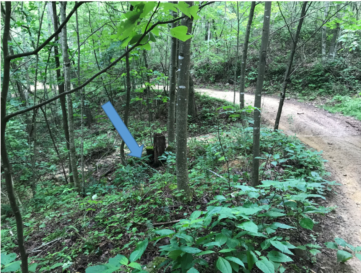
Figure 46 (Section of Trail 16 with a cut allowing unfiltered runoff from the trail to discharge over the slope into a drainage swale leading to Curran Branch; 37.29801° , -81.39059° )
