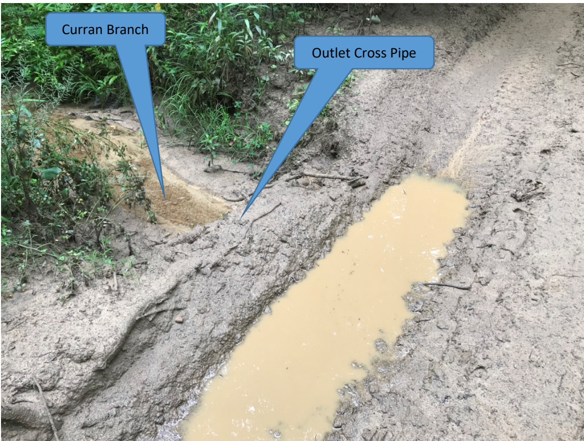
Figure 48 (Cross pipe in Curran Branch on a Section of Trail 67 and sediment deposition observed in Curran Branch from unfiltered runoff from the trail; 37.29746° , - 81.39559° )
