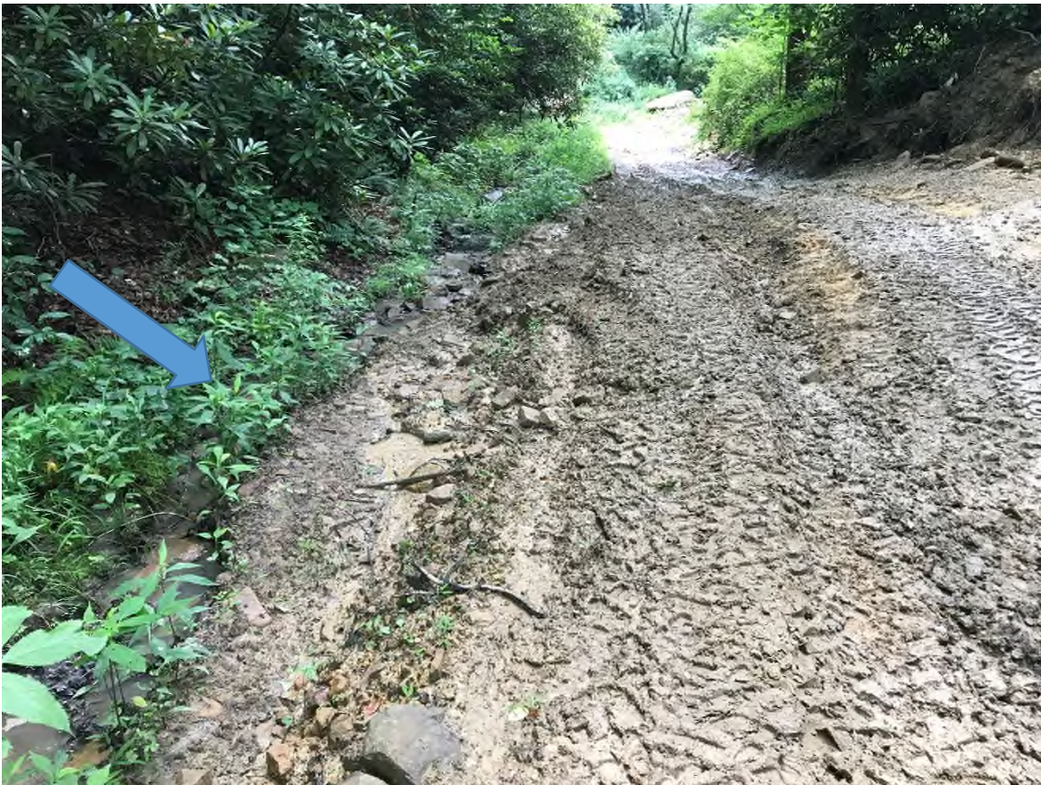
Figure 20 (Section of Trail 14 paralleling Haynes Branch with sediment deposition observed within Haynes Branch; 37.29521° , -81.37177° )
