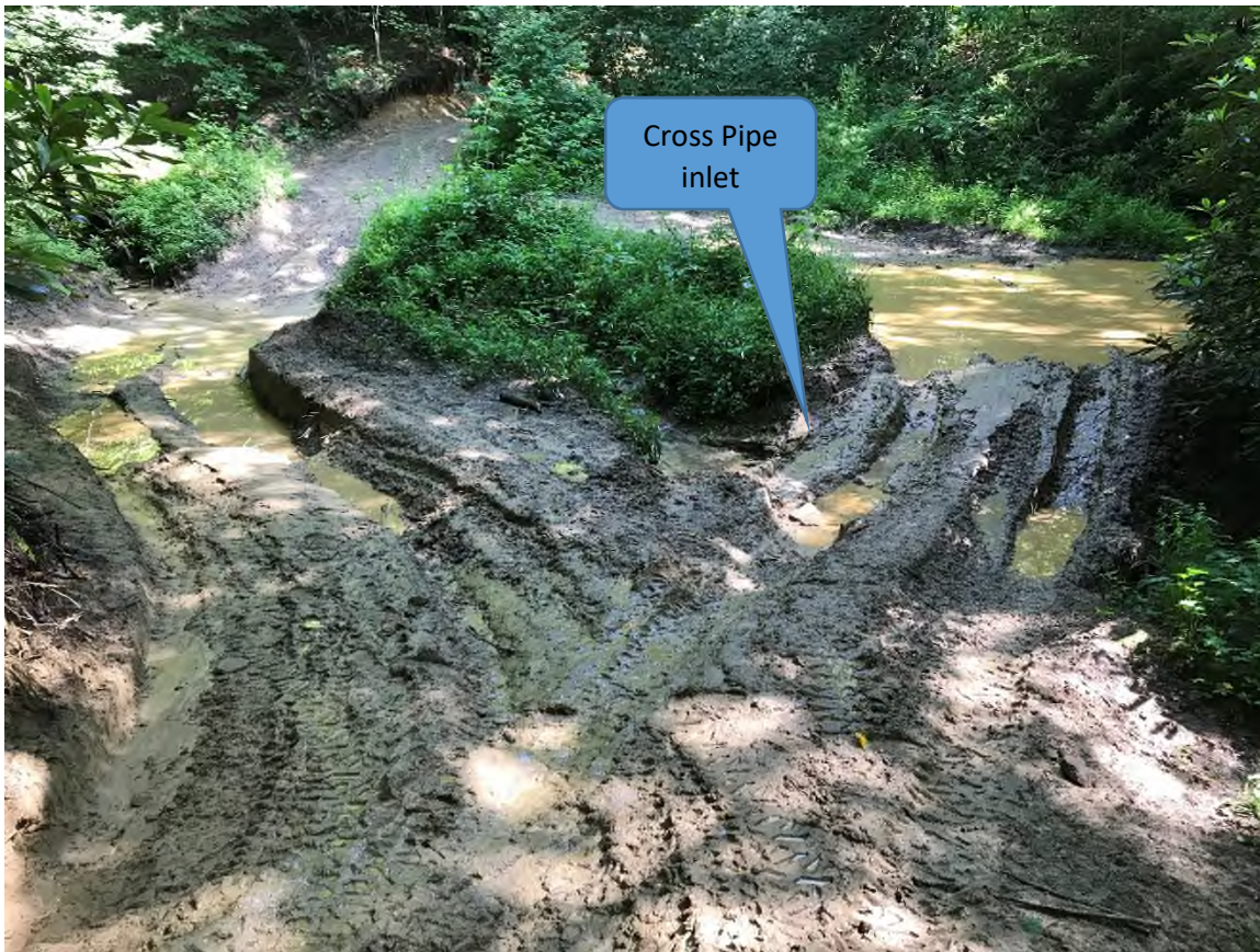
Figure 12 (Sediment deposition observed in unnamed tributary of Laurel Fork downstream of cross pipe at Trail 16 crossing; 37.29957^\circ , -81.38358^\circ )
