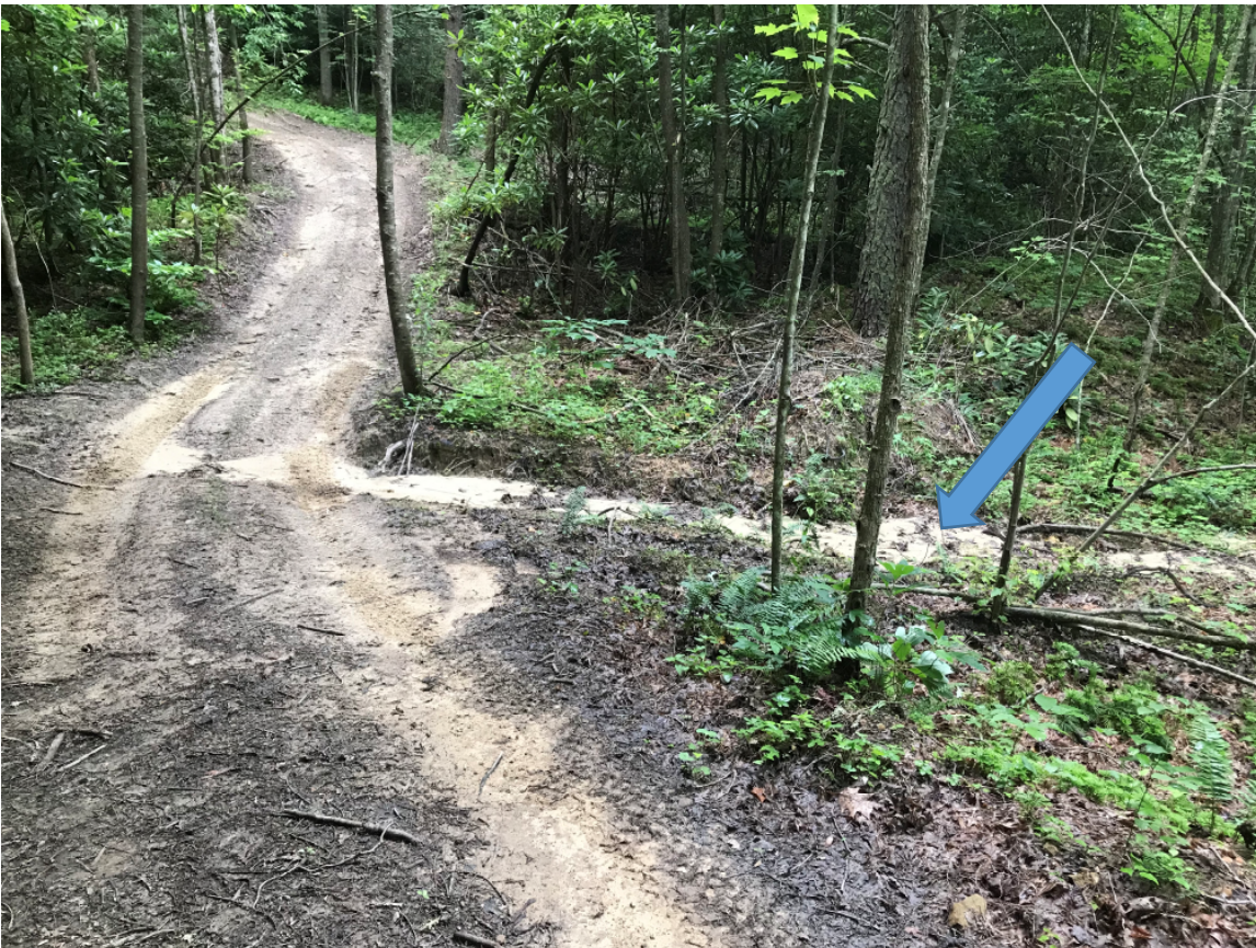
Figure 56 (Section of Trail 67 with a cut allowing unfiltered runoff from the trail to discharge over the slope into a drainage swale leading to Curran Branch; 37.29464°, -81.39353° )
