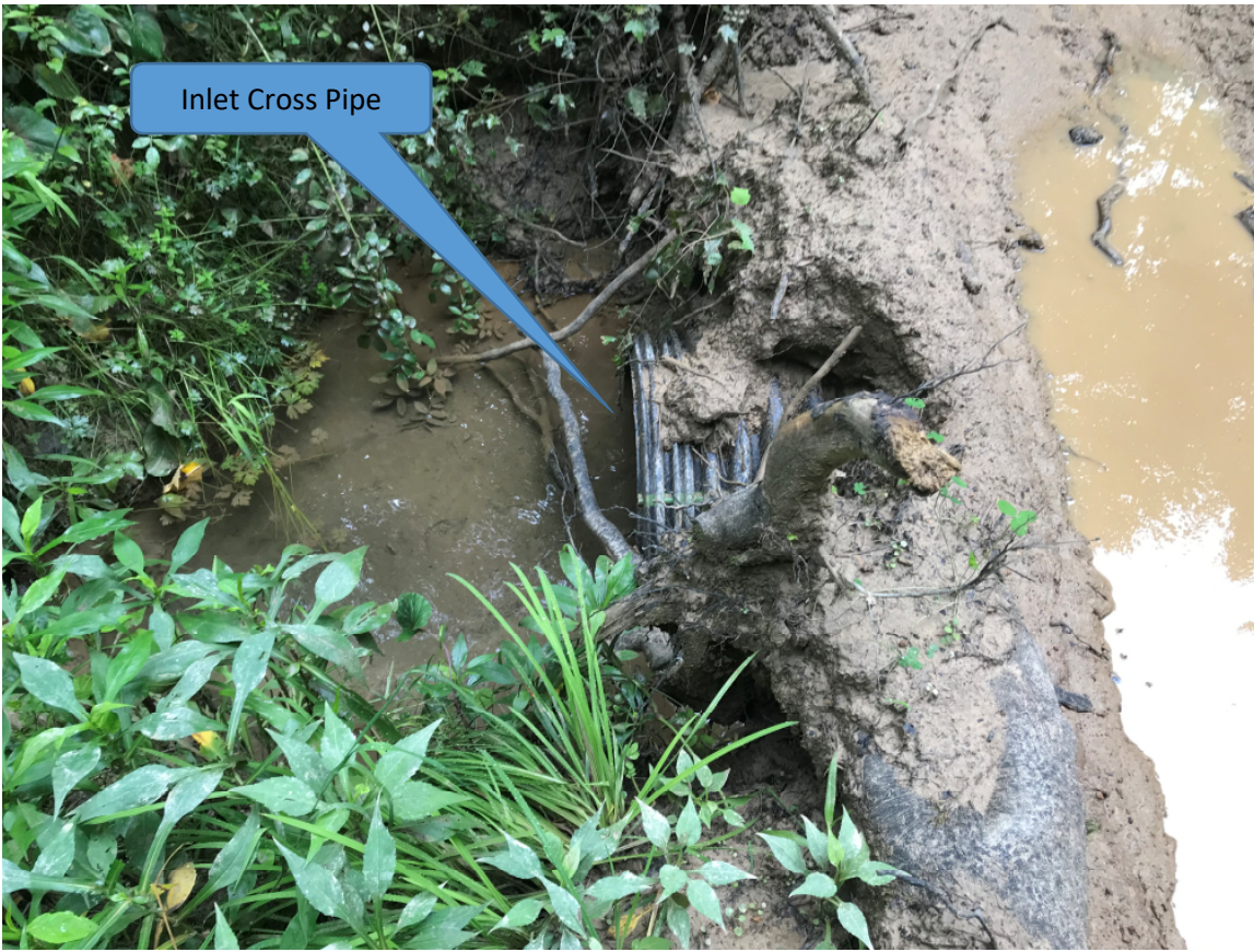
Figure 52 (Cross pipe in Curran Branch on a Section of Trail 16 and sediment deposition observed in Curran Branch from unfiltered runoff from the trail; 37.29664°, -81.39494° )
