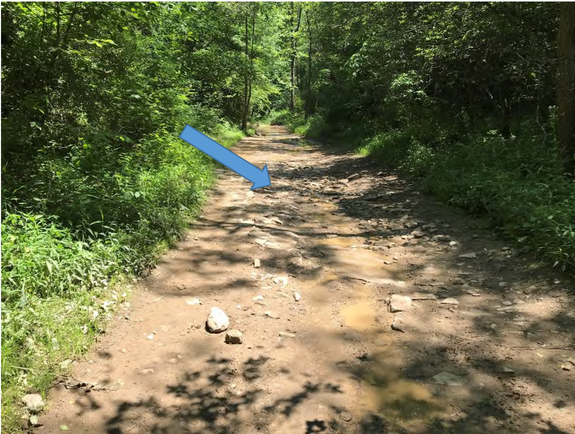
Figure 44 (Section of Trail 16 with a cut allowing unfiltered runoff from the trail to discharge over the slope into a drainage swale leading to Curran Branch; 37.29713° , -81.39059° )
