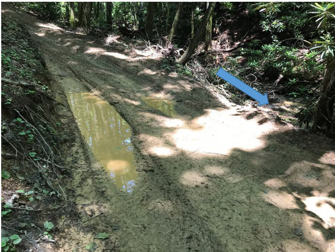
Figure 36 (Sediment from Trail 44 erosion observed discharging into Haynes Branch; 37.30516° , -81.37922° )
