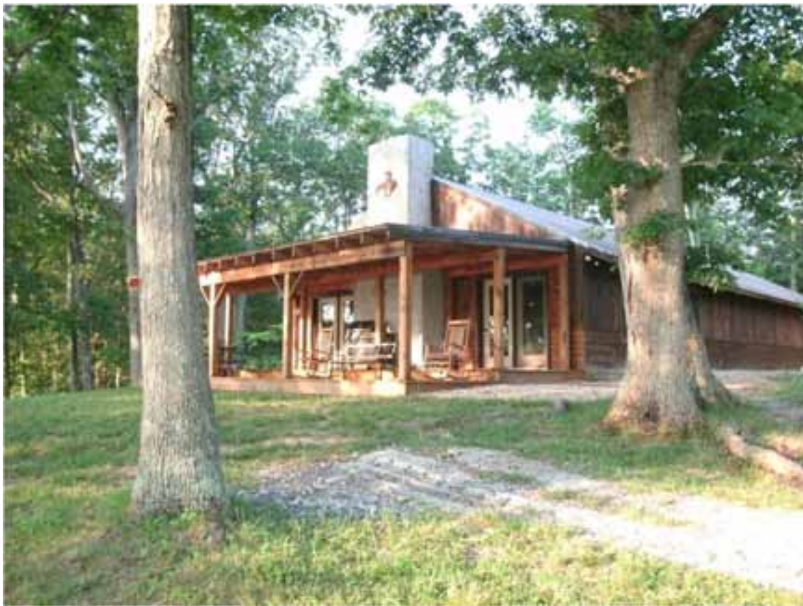
Figure 6.4: Photos of North Mountain Outfitters Bunkhouse
